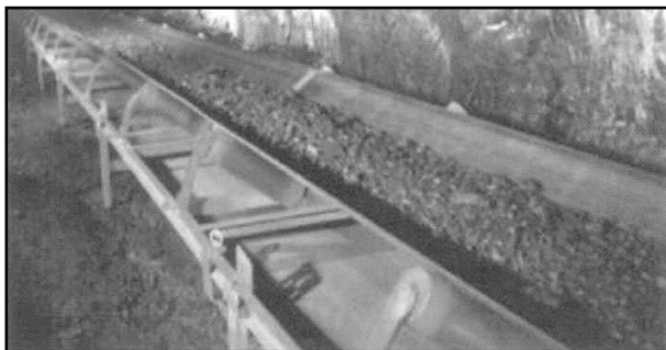
Example of a typical belt conveyor
